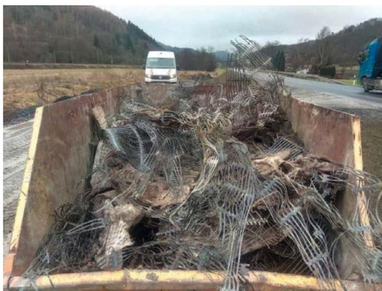
**Fig. 2:** Deconstructed geogrid and nonwoven fabric in skip
