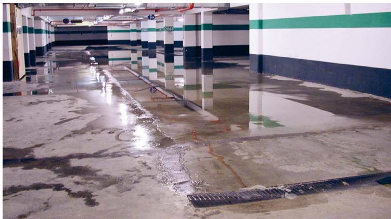
**Fig. 2:** Leaking cracks in the floor slab of a parking level
