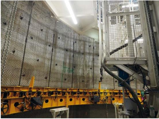
**Fig. 20:** Freeze shaft showing the very stable freeze wall
