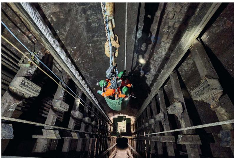
**Fig. 1:** Descent being made by bucket to the mobile working stage in Konrad 1 shaft, 2018
