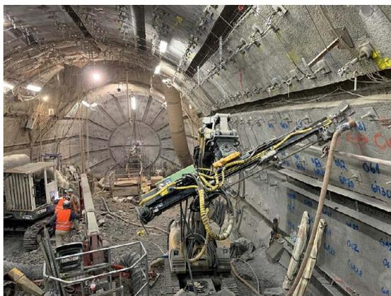
**Fig. 5:** One of the main advantages of shotcrete is flexible adaptation to the geometry of the spraying surface.
