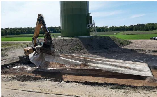
**Fig. 4:** "Pulling free" the geosynthetic layer with sorting grab
