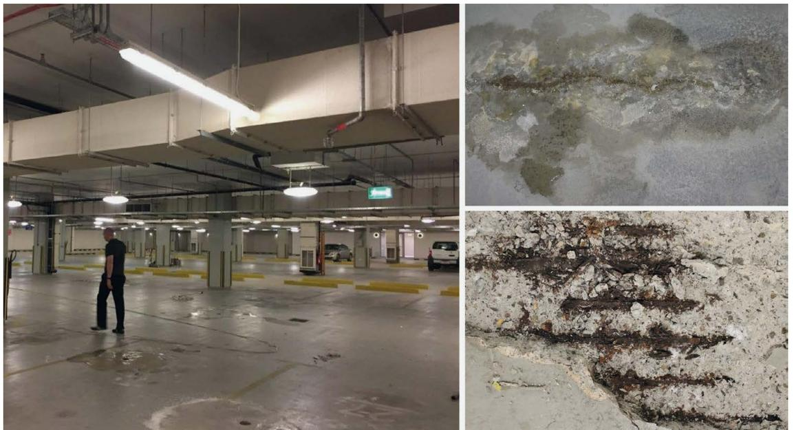
**Fig. 6:** Floor slab of an underground car park in the United Arab Emirates with non self-healing water-bearing cracks and heavily corroded reinforcement
