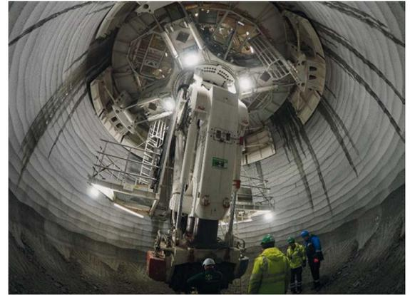
**Fig. 21:** Significant agglutination problem in the calcareous formations mainly affected the suction system.
