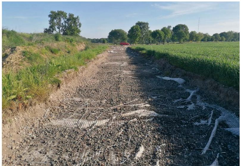
**Fig. 1:** Exposed sub-base reinforcement of a temporary access road
