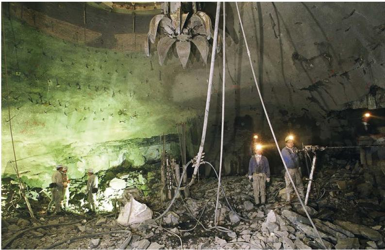
**Fig. 11:** Excavating the shaft landing on level 7 – external support system with grouted anchor bolts and dry-sprayed shotcrete
