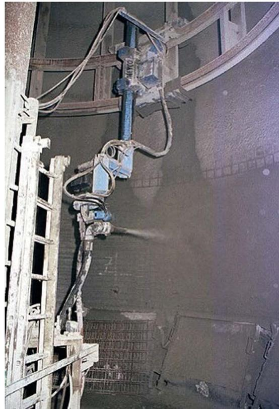
Fig. 6: Using a manipulator to apply shotcrete
