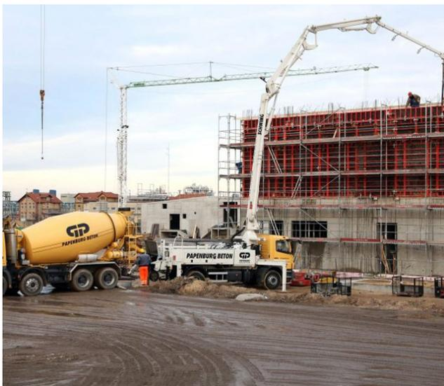
**Fig. 1:** Structural engineering projects usually allow other work to be carried out while concreting is under way.
