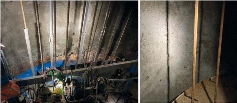
**Fig. 15:** Cramped shaft conditions (left) and the final result of the concreting operation (right)
