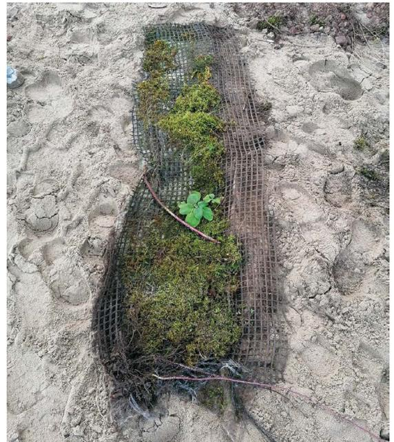
**Fig. 5:** Overgrown geogrid and nonwoven from the facing of a reinforced-soil structure
