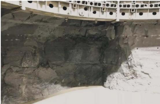
**Fig. 22:** Collapse directly below the formwork support ring
