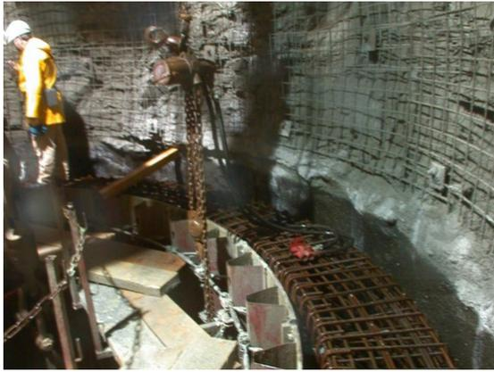
**Fig. 3:** Cramped site conditions for the concrete formwork
