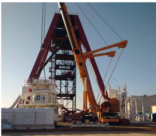
Fig. 18: View of shaft before the scaffold is lowered into place – the concrete distributor is in the left foreground
